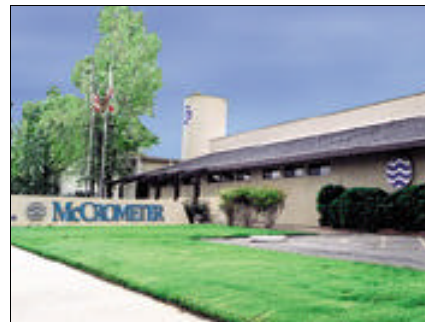
McCrometer's Company Headquarters in Hemet, California
